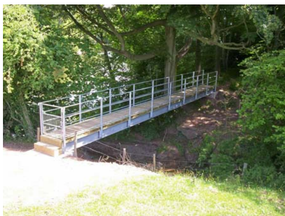
New Bridge on the Maelor Way
