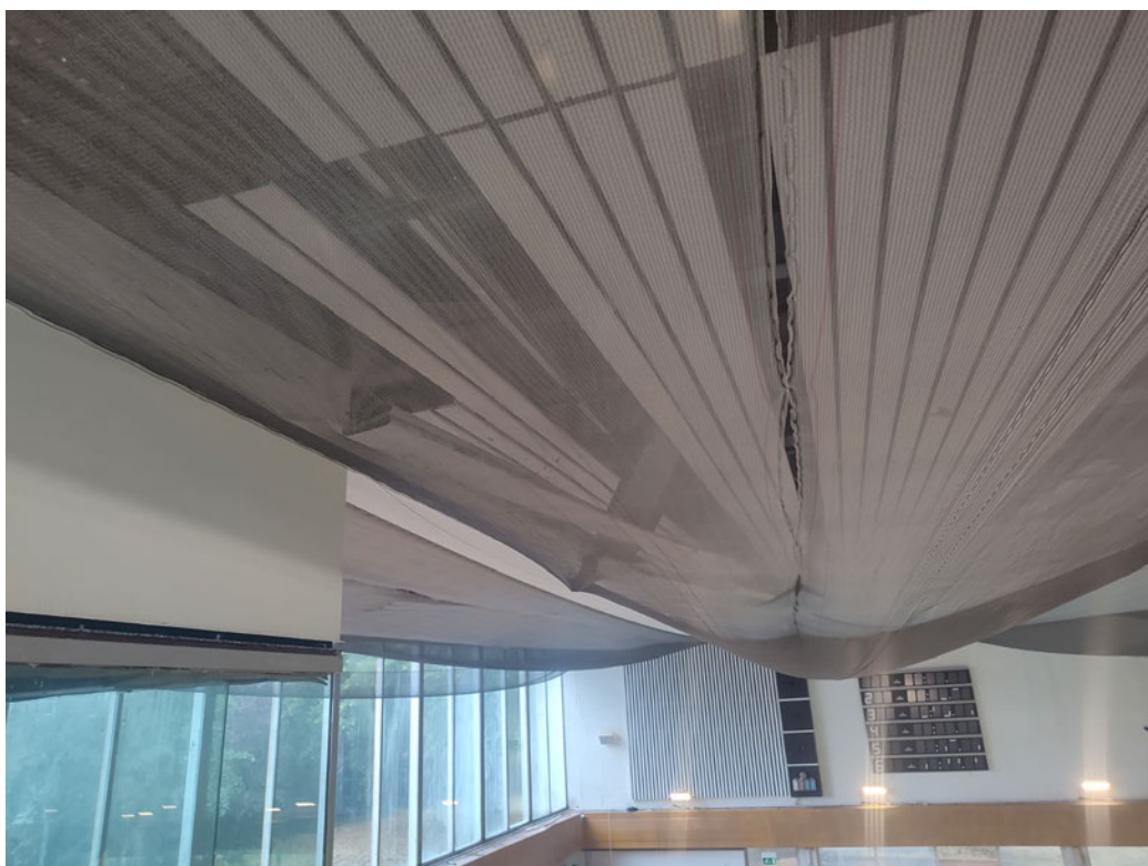
Safety netting beneath light weight ceiling slats
