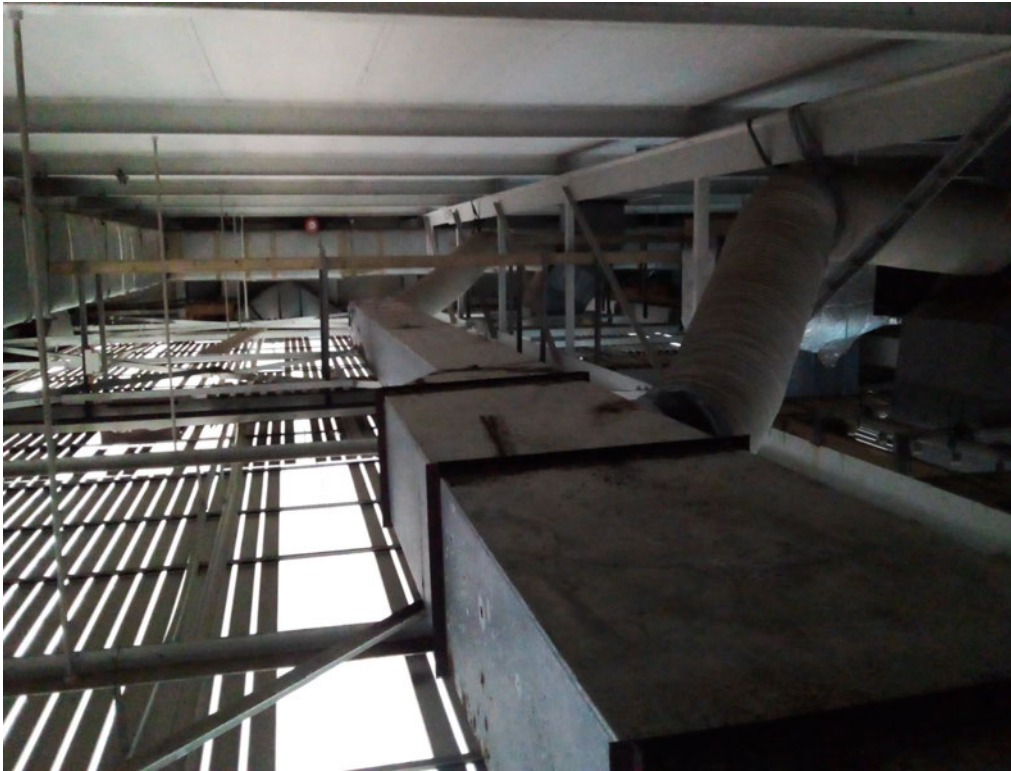
Ducting, suspended ceiling, walkways flexi hoses to be removed
