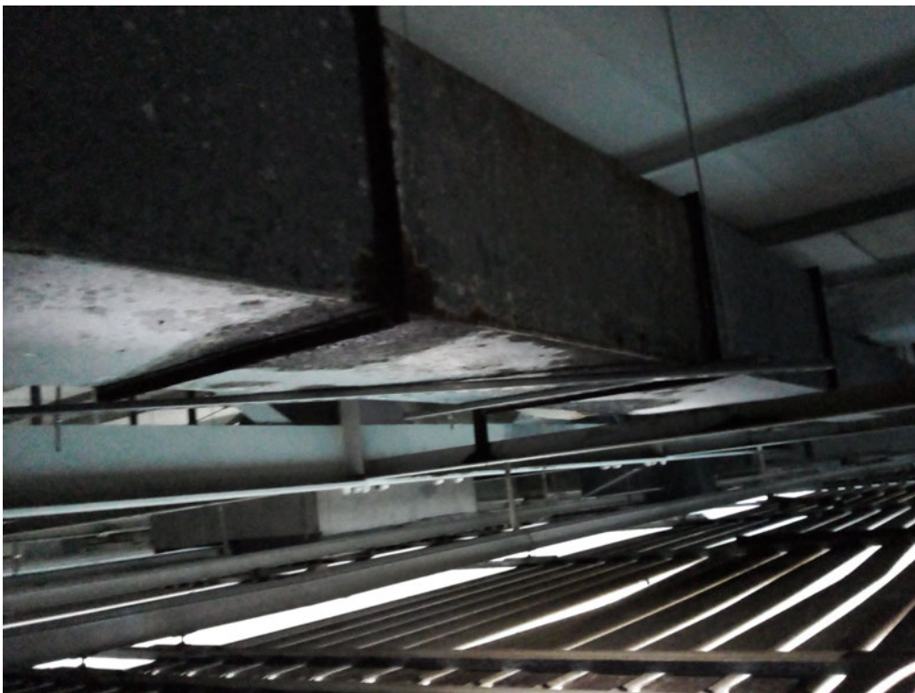
Typical ductwork section, suspended from flange clamps with threaded bar
