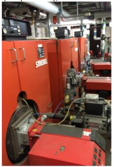
All the centre heating provision is by a primary hot water circulation system serviced by three strebel gas fired boilers that have relatively new burner heads and are in good condition for their age. Although they are not as energy efficient as newer boilers they are moderated by an automatic operating sequencer, which improves their efficiency and they remain serviceable.
