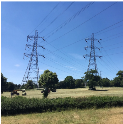
1. FROM B4373 NEAR DUNGEGROVE FARM LOOKING ALONG OVERHEAD LINE TO THE WEST
