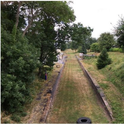
1. FROM MINOR ROAD, VIEW SOUTH EAST ACROSS FORMER RAILWAY PLATFORMS
