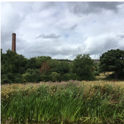
3. THE CHIMNEY WITHIN THE LIME KILN IS VISIBLE ABOVE THE VEGETATION
