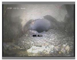
Photo: 70\_3A, Media No:: 290819\_1, 00:00:41 0.72m, Settled deposits, fine, 45% cross-sectional area loss
