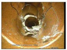
Photo: 72\_12A, Media No:: 290819\_1, 00:01:58 14.66m, Broken pipe, from 9 to 3 o'clock Remarks: Excavation required to repair
