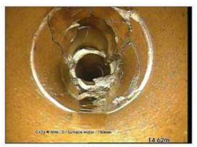
Photo: 72\_10A, Media No:: 290819\_1, 00:01:46 14.62m, Fracture, multiple, from 9 to 5 o'clock
