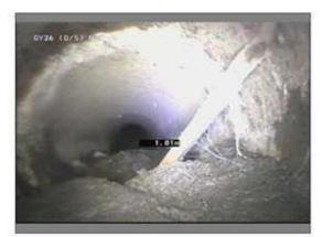
Photo: 69\_3A, Media No:: 290819\_1, 00:00:29 0.98m, Settled deposits, fine, 40% cross-sectional area loss
