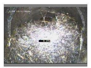
Photo: 31\_3A, Media No:: 290819\_1, 00:00:18 0.28m, Roots, mass, 60% cross-sectional area loss
