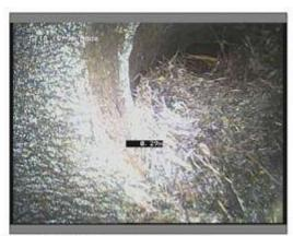
Photo: 31\_3A, Media No:: 290819\_1, 00:00:19 0.29m, Survey abandoned Remarks: Unable to pass root mass - root cutting required
