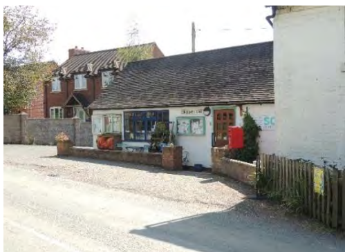
Post office and shop
