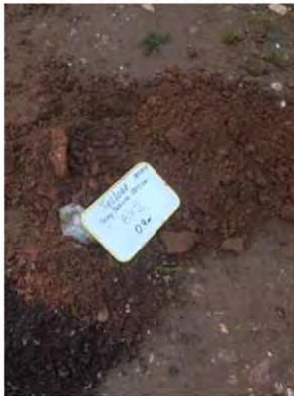
Photo 2: BH2 spoil during excavation work
