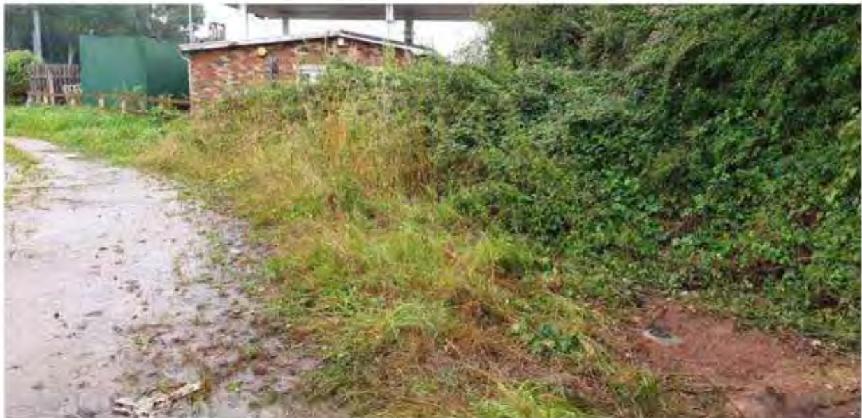
Photo 4: Location of BH1 in relation to the PFS (the canopy of the PFS can be seen in the background)
