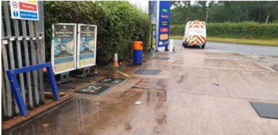
Photo 7: Fill point covers of the USTs on site
