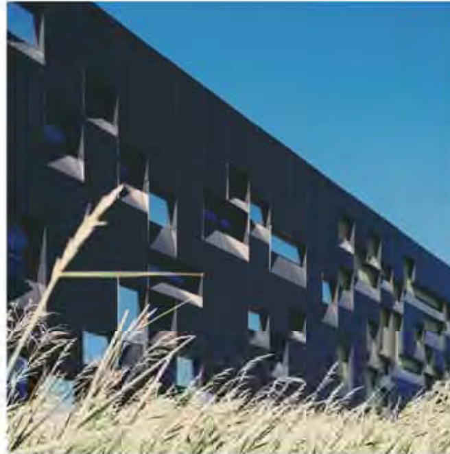
Figure 88; Bold Architecture Contributing To A Sense Of Place.
