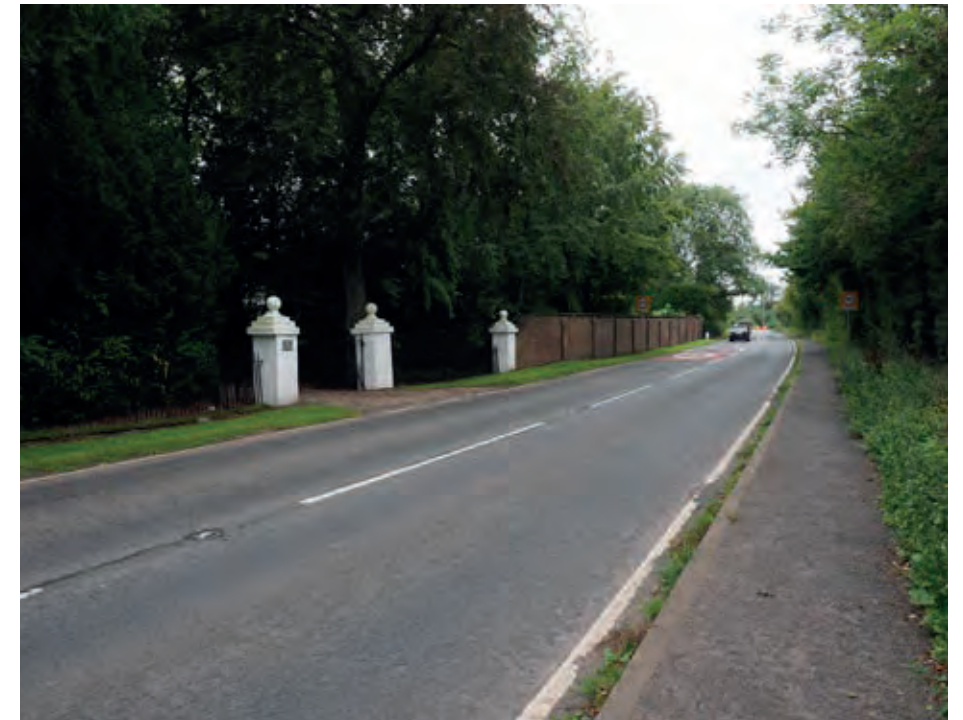
View north west along A464.
