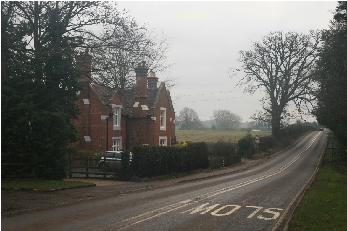
Image EDP 6: Photograph taken from Stourbridge Road westwards to the southern site boundary. Photograph was taken in January 2019. Viewpoint location is situated at SO 74188 92371
