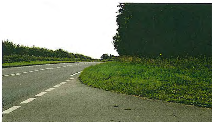
Visibility from Watling Street North Junction to the North at 2.4m
