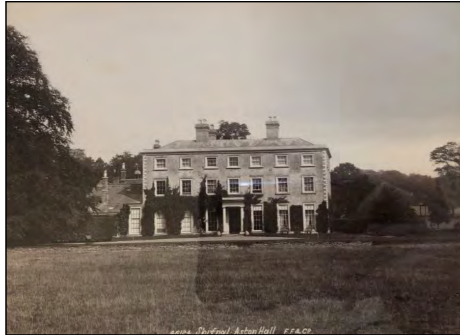
Figure 18 c.1900 photograph of the primary (southwest) elevation of Aston Hall.
