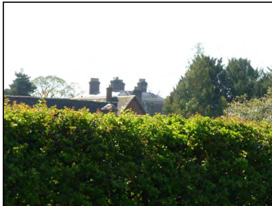
Figure 21: A partially zoomed view of part of the roofscape and a small portion of the western façade of Aston Hall from Coppice Green Lane 90 m north of the junction with the drive to Aston Court Mews
