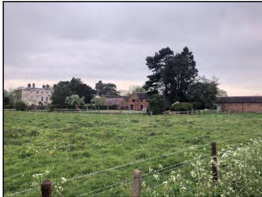
Figure 27: Aston Hall and the Barns, Byre and Hayloft, and Stables enclose the listed Water Tower and preclude views from the wider surrounds.
