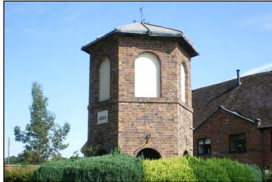
Figure 26: Water tower, approximately 20 metres to north of Aston Hall. (source: Britishlistedbuildings.co.uk)
