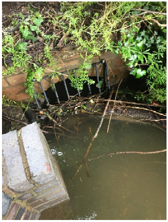
Photograph of old culvert under Poynton Road to be blocked up
