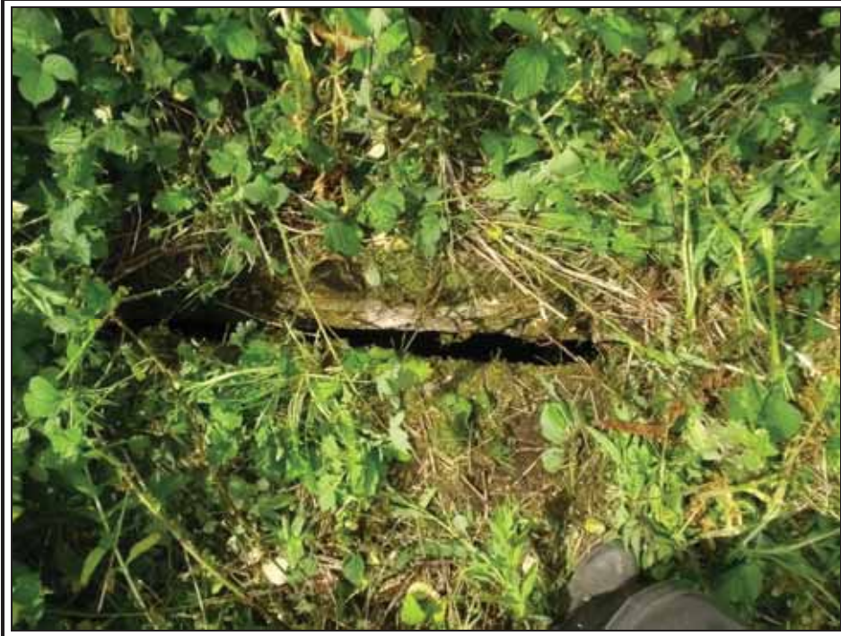
Photo 14, Hole in the top of the culvert
