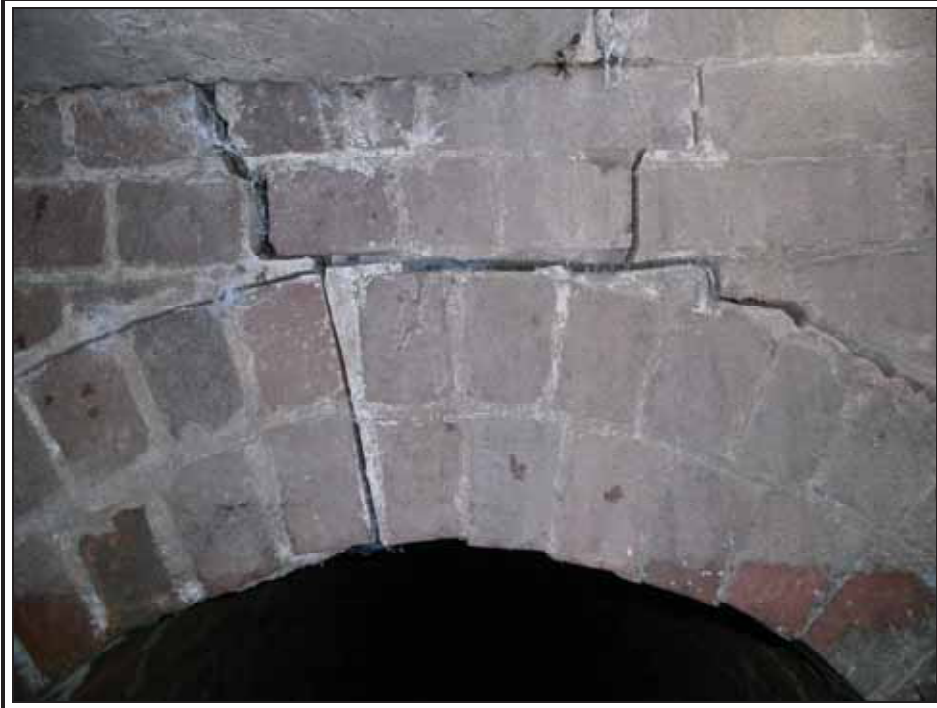
Photo 6, Defects in MH05
