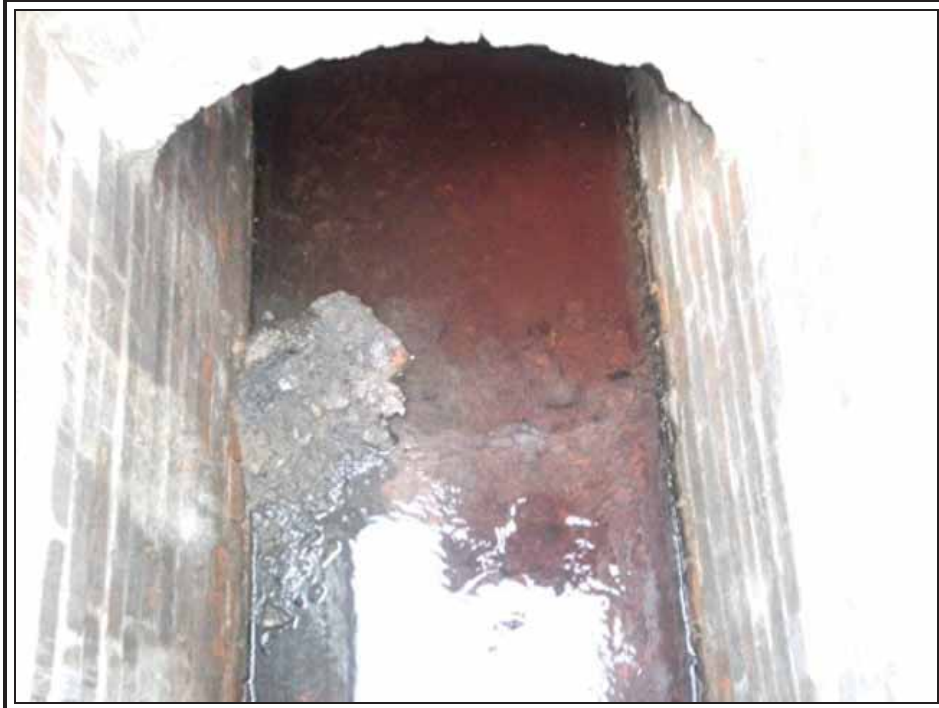
Photo 18, Tracing Dye located in manhole
