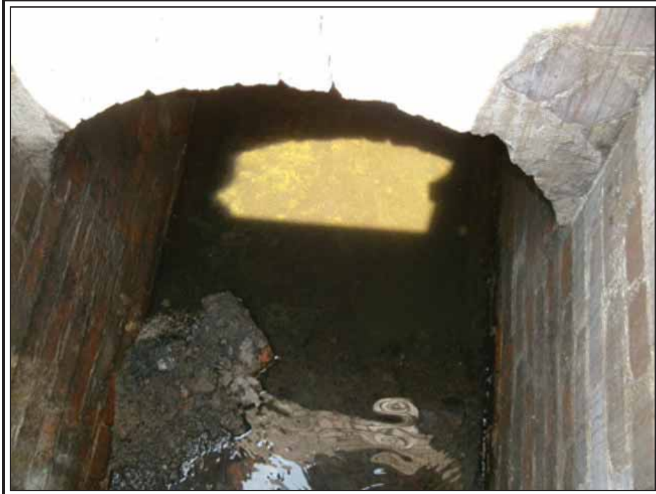
Photo 16, Evidence of foul in surface culvert in uncharted MH
