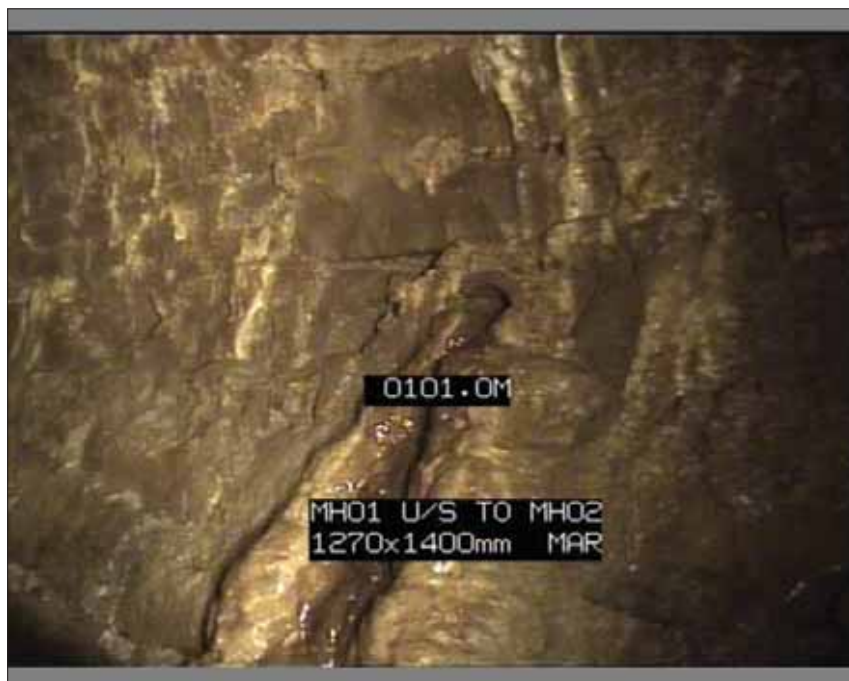
Photo: 1_24A 101m, Encrustation, medium, from 2 to 5 o'clock, 10% cross-sectional area loss
