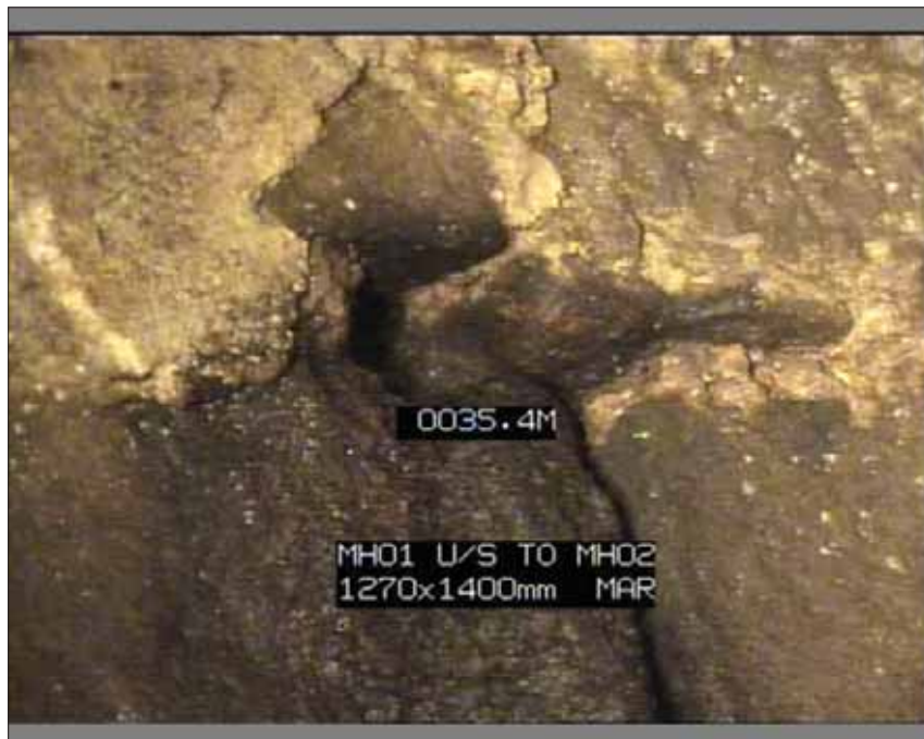
Photo: 1_11A 35.4m, Hole in sewer, at 11 o'clock
