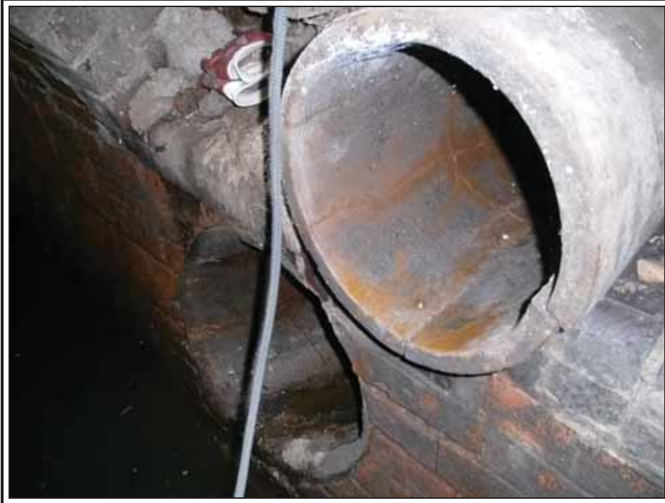
Photo 9, Overflow pipe from pumping station in MH05
