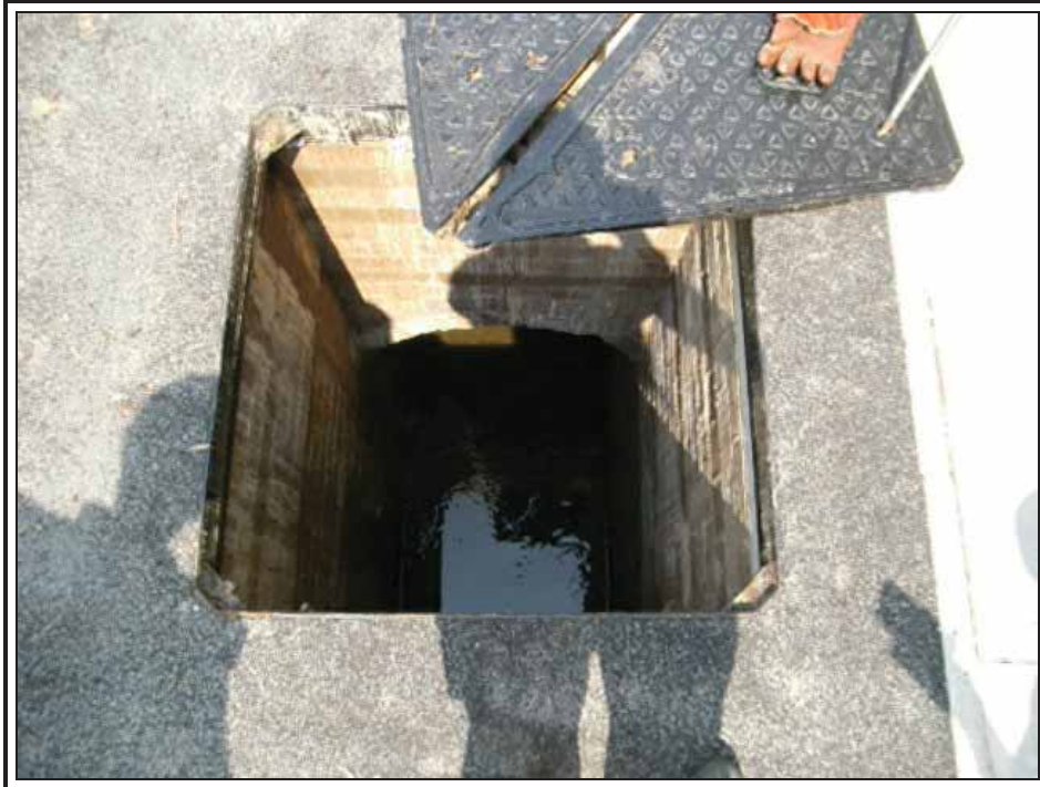
Photo 15, Evidence of foul in surface culvert in uncharted MH
