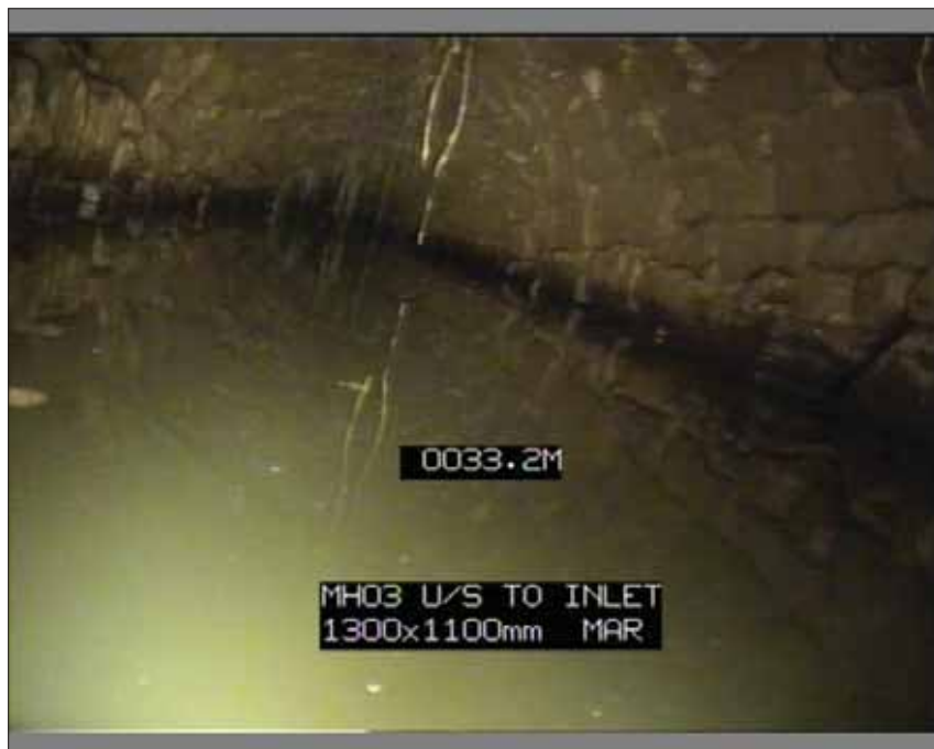
Photo: 6_10A 33.2m, General observation Remarks: Dip In Line
