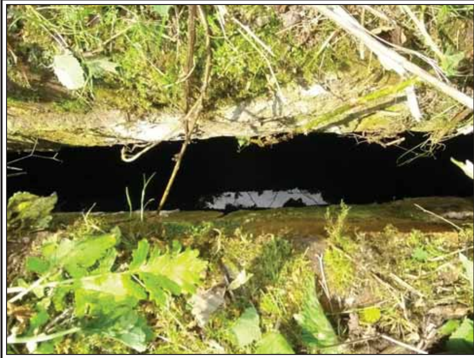
Photo 13, Hole in the top of the culvert
