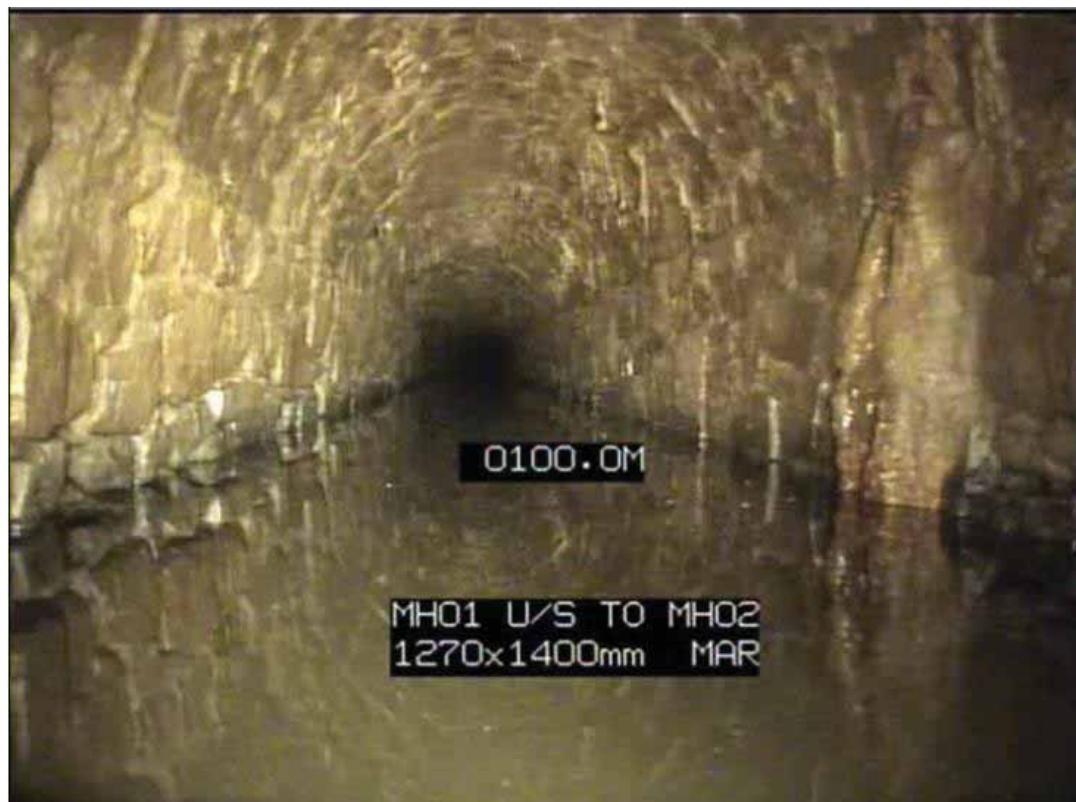
Figure 3.3 – The Typical Condition of the Tetchill Brook Culvert
