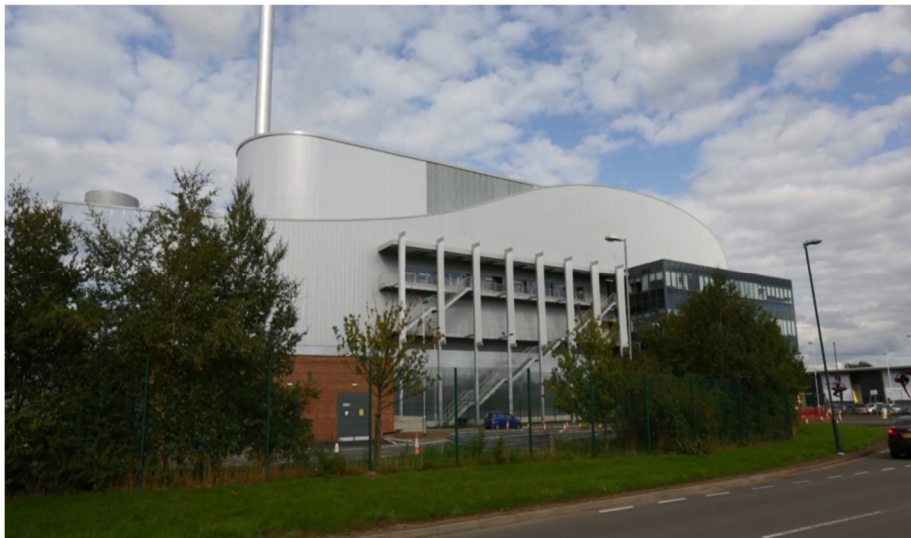
Figure 3 Veolia Energy Recovery Facility: Shrewsbury.
