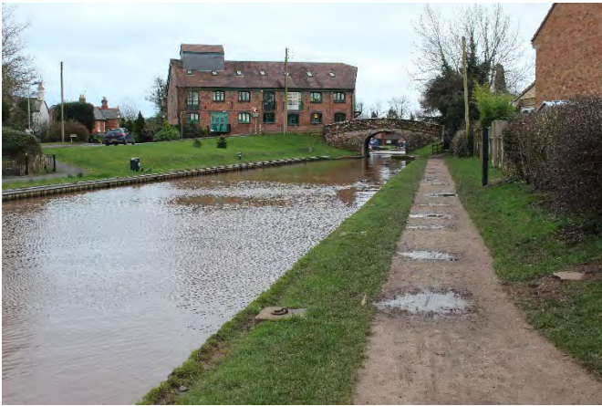
Shropshire Union Canal, Market Drayton Grove
