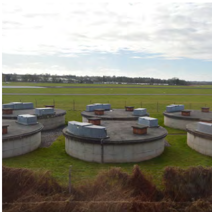
1. UNDERGROUND STORAGE TANKS, RAF COSFORD PHOTO © N CHADWICK (CC-BY-SA/2.0)
