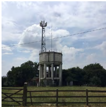
4. VIEW SOUTHWEST FROM PROW AT ST PETER AND ST PAUL CHURCH, TASLEY TOWARDS WATER TOWER
