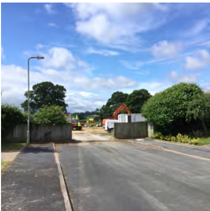
3. VIEW SOUTH FROM THE HAWTHORNS OF A PROPOSED DEVELOPMENT UNDER CONSTRUCTION
