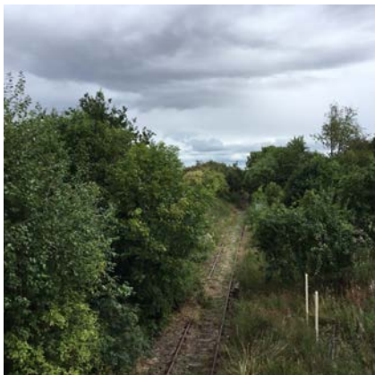
3. FROM BRIDGE OVER DISUSED RAILWAY LINE AT TWMPATH ROAD LOOKING NORTH
