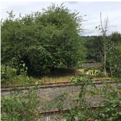
3. THE DISUSED RAILWAY LINE RUNNING ALONG THE SOUTHERN BORDER OF THE PARCEL
