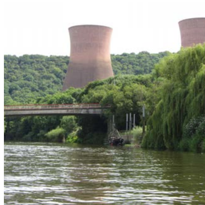
4. RIVER SEVERN NEAR COOLING TOWERS PHOTO © GARETH JAMES (CC-BY-SA/2.0)
