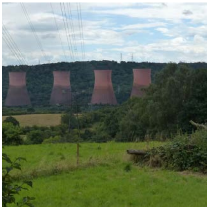
3. COOLING TOWERS FROM EDGE OF TIMBER WOOD PHOTO © MAT FASCIONE (CC-BY-SA/2.0)
