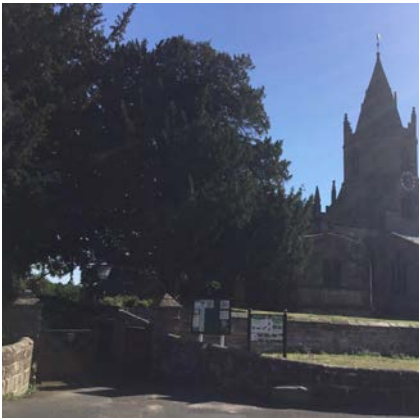
1. VIEW OF ST. BARTHOLOMEW'S CHURCH FROM WITHIN TONG
