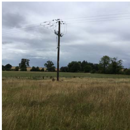
4. FROM PROW, VIEW NORTH EAST
