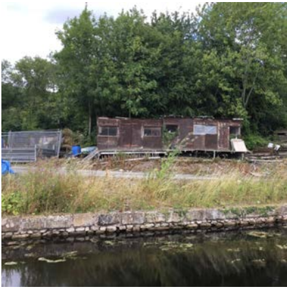
1. DEGRADED LAND IS A DETRACTING ELEMENT WITHIN THE CONSERVATION AREA
