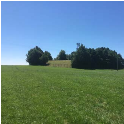
1. FROM PROW, VIEW NORTH OF THE COVERED RESERVOIR AND MAST AT A HIGH POINT IN THE
