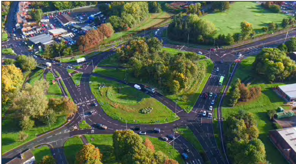
Traffic, pedestrian and cyclist improvement at Meole Brace Island
