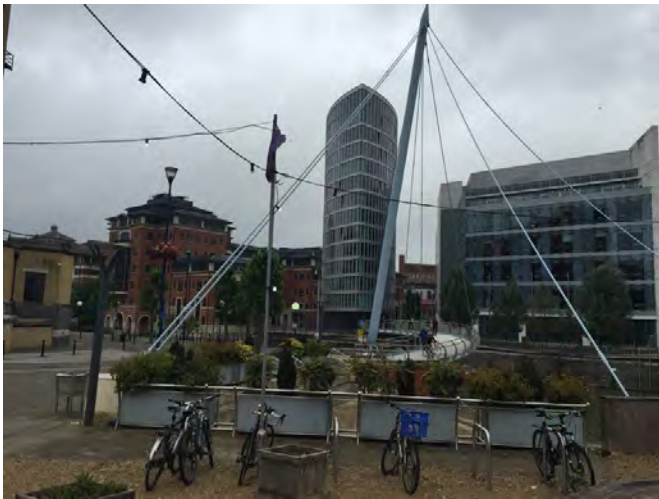
Valentine Bridge: landmark curved foot/cycle bridge as a feature of new development near Temple Meads Station/Enterprise Zone
