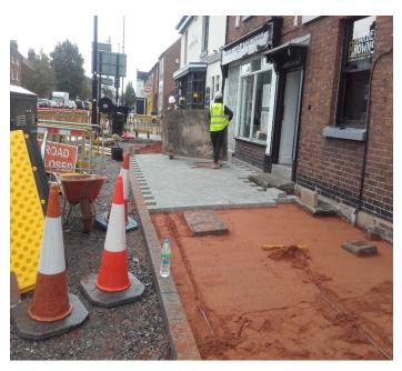
Old kerbs and pavers were excavated and taken to a transfer station where they will be recycled for re-use.
