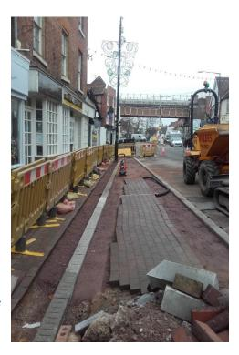
The new drain has been connected to the existing drainage system. Works in this location have been made safe with tarmac as a temporary measure to allow footways to be re-opened to full width and allow unhindered access to the shop fronts during the Christmas embargo period\*
