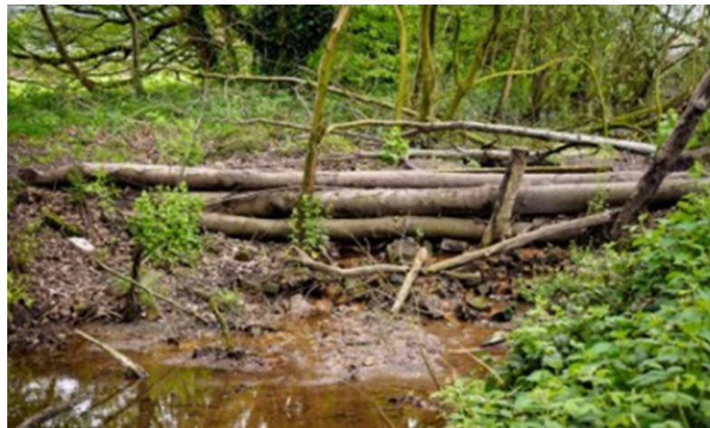
Figure 6: Traditional NFM structures, such as leaky barriers, can be used to enhance channel-floodplain connectivity to encourage pollutant deposition.
