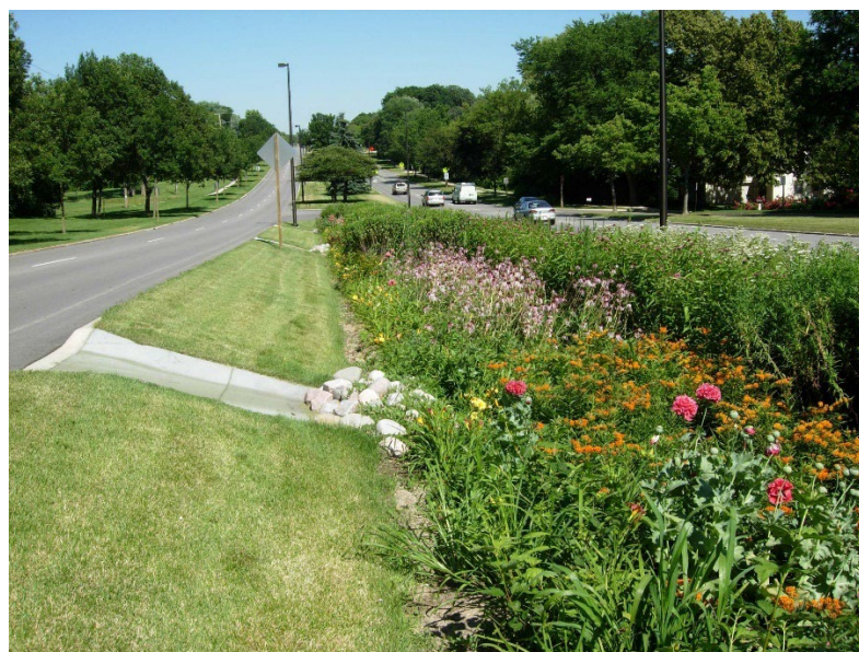
Figure 11: Example of a bioretention zone (Source: Welshwildlife.org)
