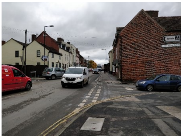
Figure AB.24 Tenbury Road junction illustrating lack of pedestrian footways
