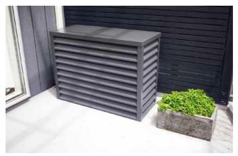
**Figure 74:** Air source heat pump housing covers the unit and harmonises with the building aesthetic
