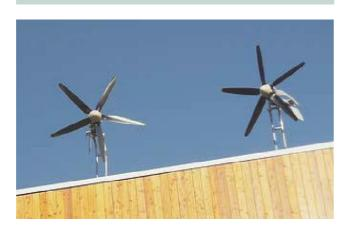
**Figure 67:** Micro-generation wind turbines can be discreetly applied on top of roofs
