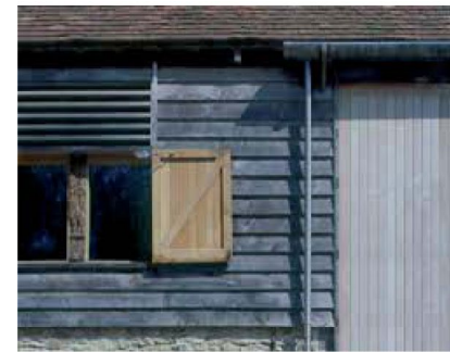
Contemporary timber shutter set within cladding
