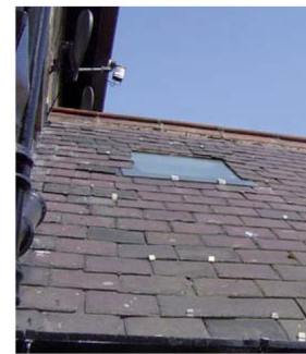
Slate roof with in-line glazing.
