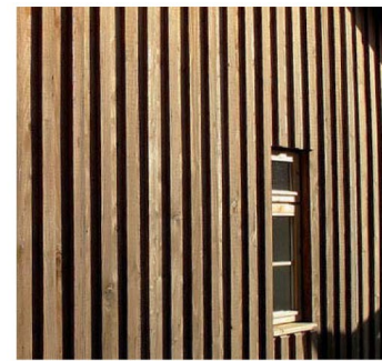
Vertical Timber Cladding
