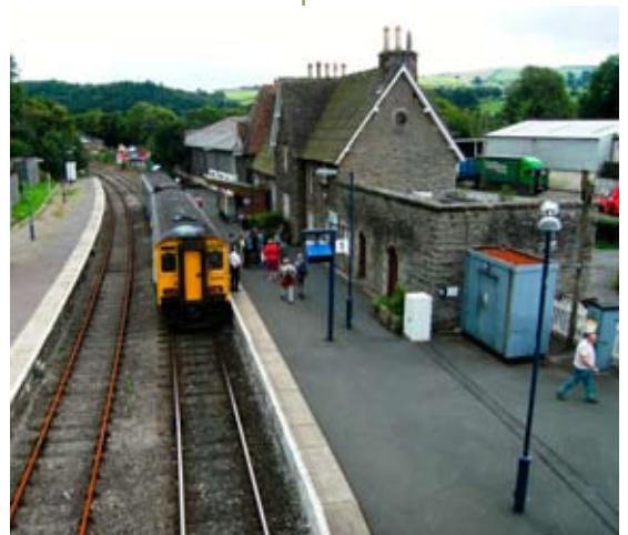
Three railway routes offer opportunities for sustainable travel in the AONB (Knighton station)
