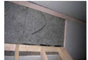
Sheep's wool insulation in renovation of an old cottage
