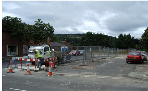
Figure 8.6: Former Castle Street Garage
