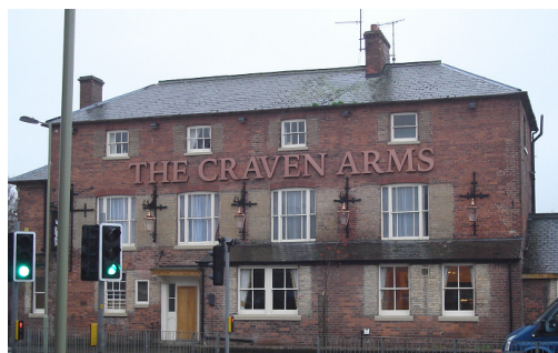
Figure 4.32: The Craven Arms public house
