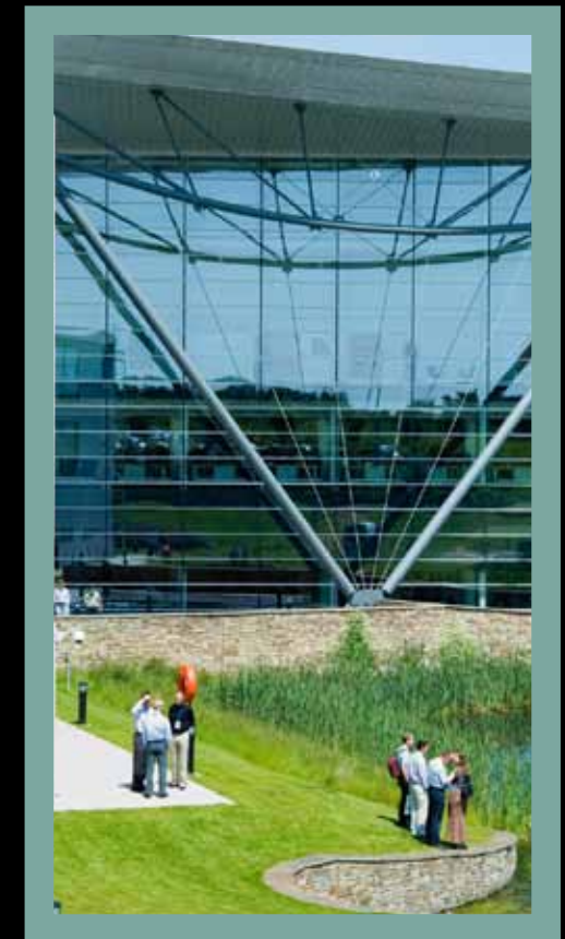
Sustainable office: The Met Office
