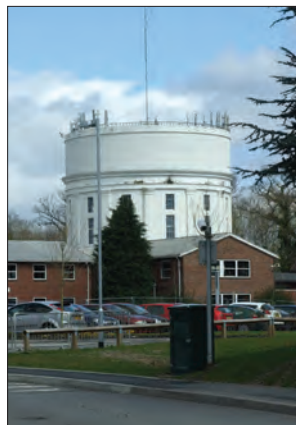
Water Tower of Severn Trent Water works.
