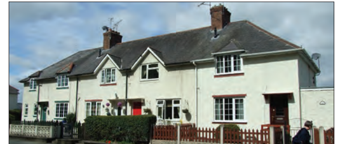
1920s housing arrangement at Shelton Gardens.
