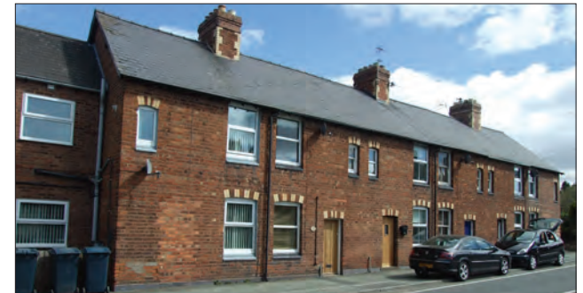
Terrace of Victorian houses on Welshpool Road.
